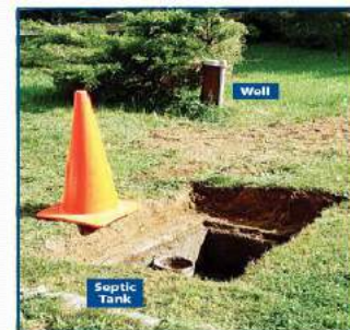
Figure 7: Well too close to septic tank – well/trank should be at least 15 metres (50 feet) apart
