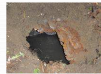
Steel Barrel Being used as a Septic Tank
